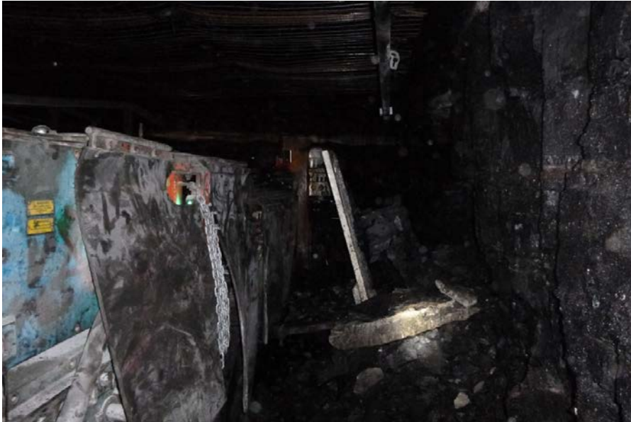
Figure 3 – Rib failure striking platform. Note that the platform has been rotated back down towards the normal operating position (SinNot-2018/00854). Photo courtesy of the mine.
