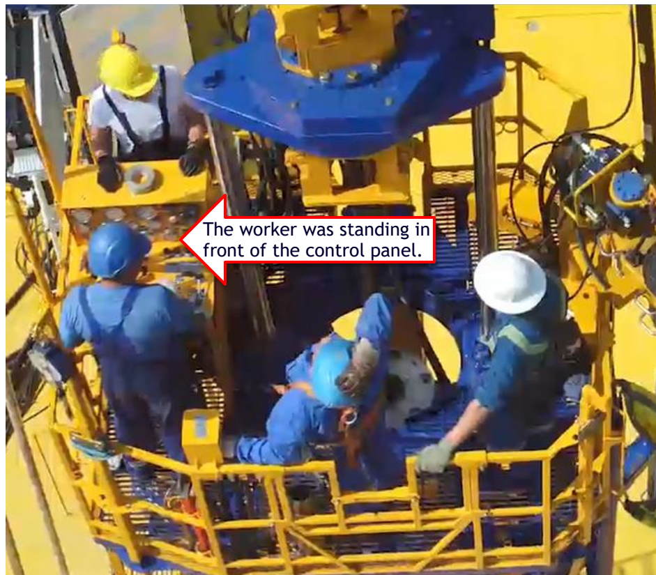
TYPICAL SET-UP OF A WORK PLATFORM ON A SNUBBING RIG. THE WORKER WAS STANDING IN FRONT OF THE CONTROL PANEL WHEN THE INCIDENT OCCURRED.
