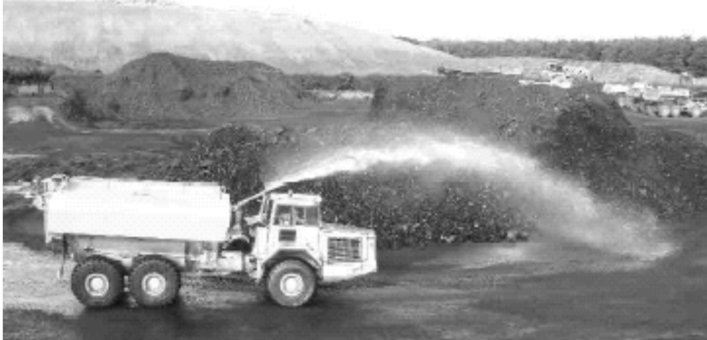
Dust suppression on stockpiles
