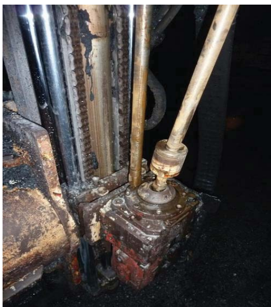
Failure of the gripper jaws to support the drill string leads to a serious hand injury
