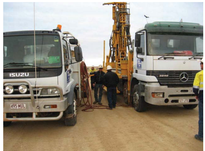
Refuelling pod mounted on support vehicle
