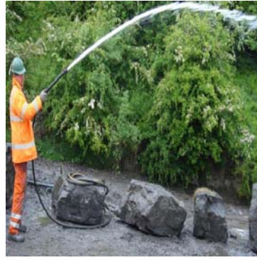
Picture 2: Pump Working
