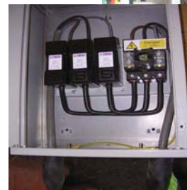
New panel with IP2X protection
