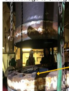
Slip flange – note bolts assumed to be securing sections
