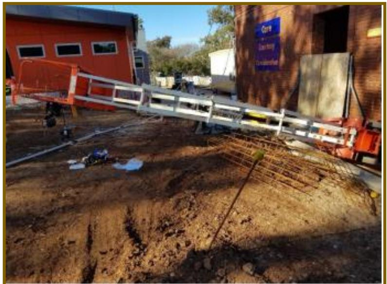
The weight and momentum of the conduit contributed to the MEWP to tipping over with both workers inside. Both workers suffered spinal fractures and one worker a fractured eye socket.
