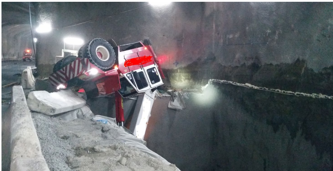
Photo: 25t Terex articulated mobile crane on the edge of 10m deep shaft
