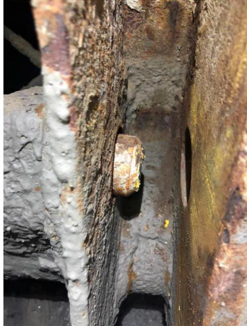
*Figure 4. Gouge marks on face of workbox locking pin receptacle*
