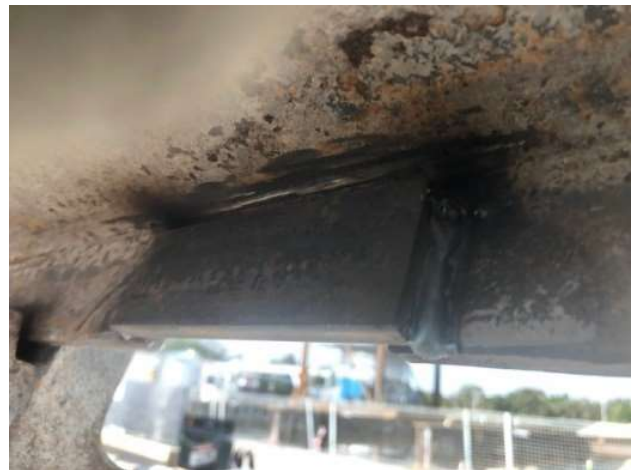
Fig 2. Plate welded to plant
