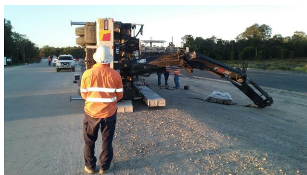
Post event re-enactment showing position of operator during the lift.
