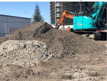
Excavator involved in the incident and the depression in the stockpile is where its' bucket dropped.
