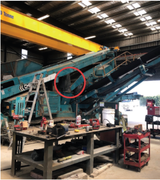
Figure 1: Worker lost footing to the right of the ladder making their way along the mobile plant
