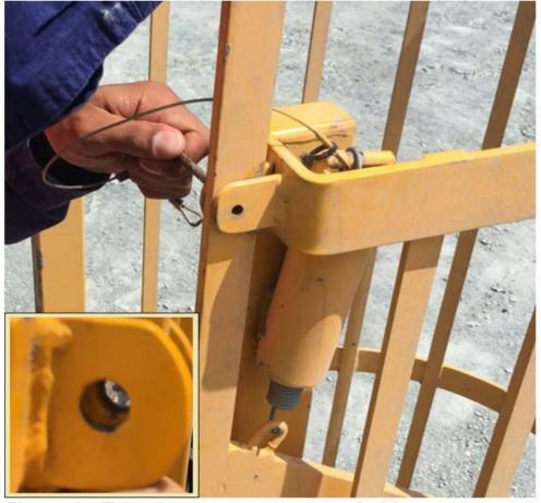
Figure 6 - Top of emergency escape ladder near operator's cabin. Misaligned holes caused the release pin to be stuck. The inserted photo is from a similar machine at another mine site, also showing misalignment. Note the undercut bracket welding
