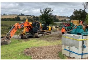
A contractor was engaged to remove an 18m x 1050mm casing from a trench using a winch truck. The rope was rigged to an excavator through a snatch block to the casing, and then through a second snatch block and anchored to the excavator.
