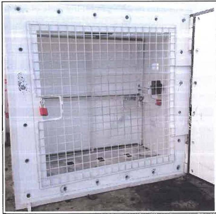
Figure 2: Hatch Seal fitted with a lockable mesh barrier
