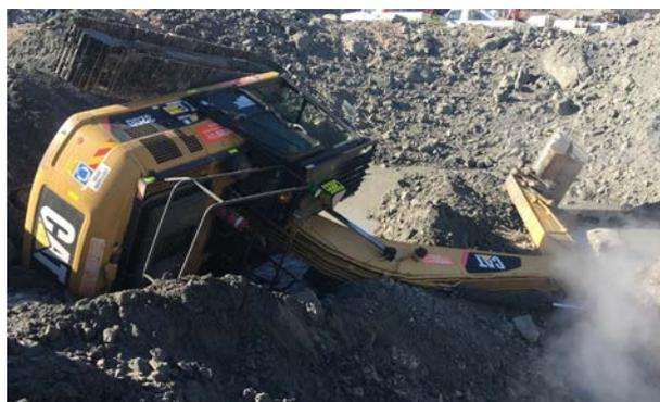
When working near heat-affected ground, the ground stability needs to be considered when preparing a safe work procedure.
