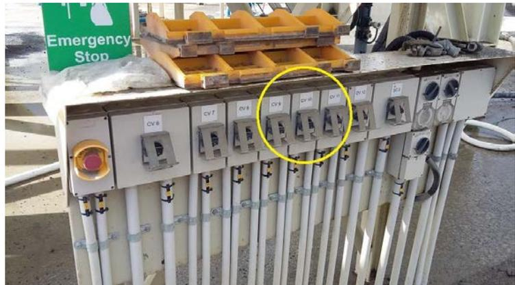
When he noticed no material on the belt he investigated to find that the locked-out conveyors had not started, and a considerable amount of material had built up at the transfer point between the feed belt and the isolated conveyors.
