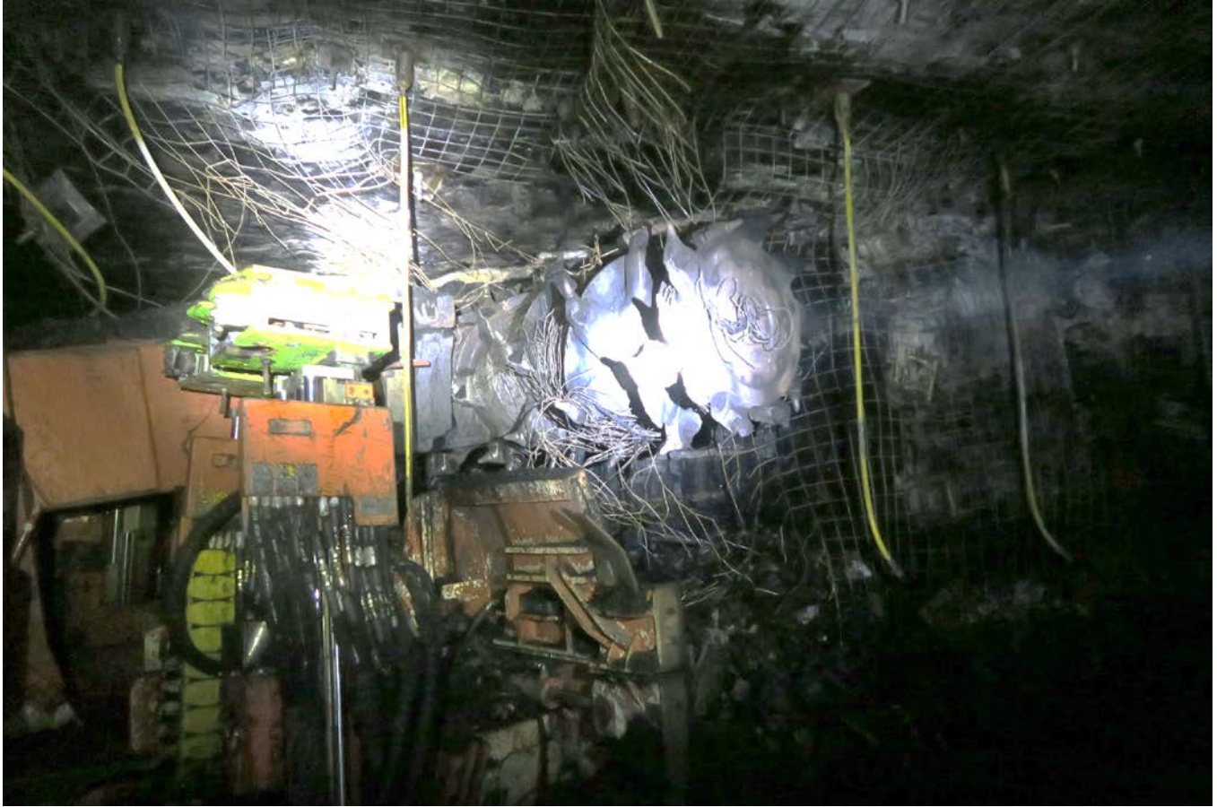
Photo 2: Continuous miner showing cutter heads and entangled rib mesh and bolts. Picture by Resources Regulator investigators.
