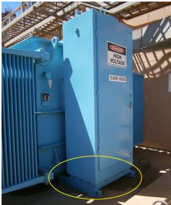
Left: High-voltage transformer, indicating where the gland plate was located on the inside base of the transformer's junction box. Right: Damaged gland plate.
