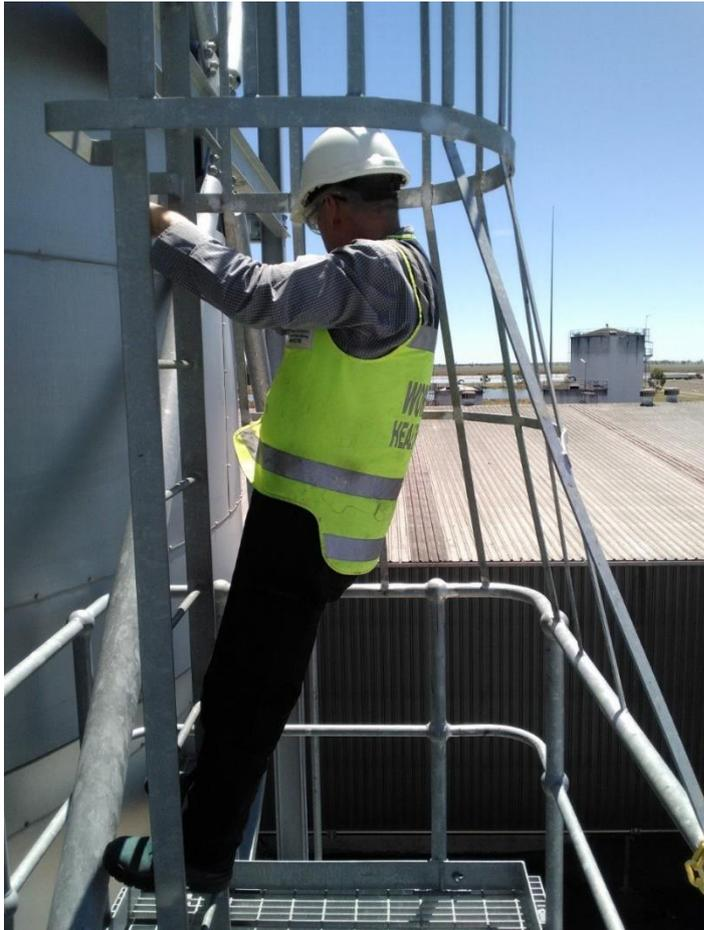
Photograph 2. The bottom of this vertical caged ladder has been flared out and extended down to the top guardrail.
