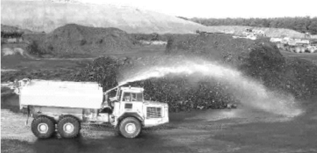
Dust suppression on stockpiles
