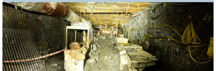
Mining tunnel where the fatal outburst occurred.
