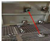
Cardoxing porthole flange removed to gain access to retrieve the over inserted Cardox tube
