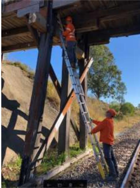
**Figure.1** Ladder footed, 3 points of contact and 4:1 ratio
