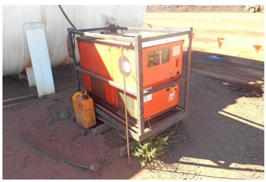
Poor housekeeping standard at a temporary generator installation.
